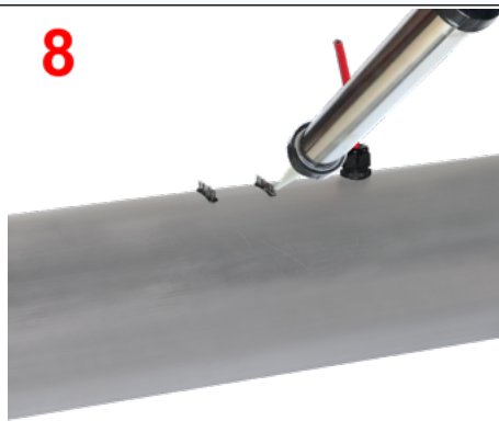
8: Inject sealant around the legs
